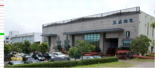
AWEA Headquarters / 26,000 m 2
