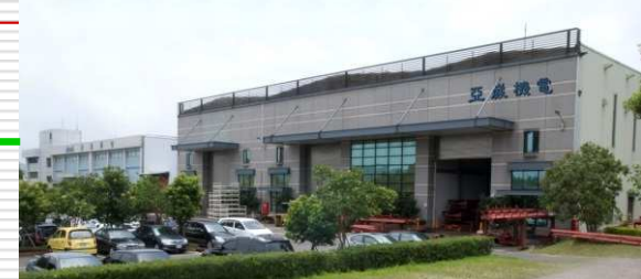
AWEA Headquarters / 26,000 m 2
