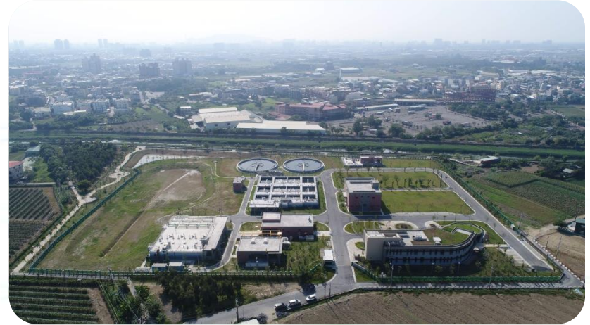
Gang-Shan Sewage Treatment Plant
