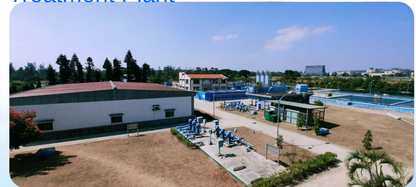
King-men Tai Lake Water Treatment Plant
