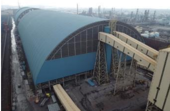
CSC New Coal Enclosed Building Conveyor System, renovation work, Ph. 2 Project
