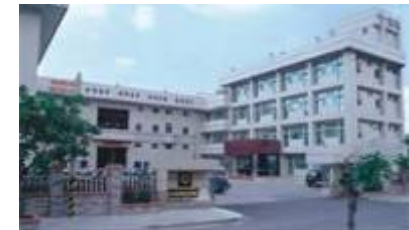
TY Machining & Welding Factory (5,200 m 2 )
