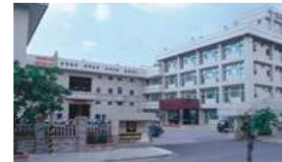
Tsang Yow Cheng-gong plant, TAIWAN (5,200 m 2 )
