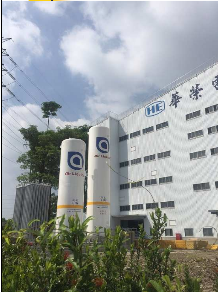
Replace fuel-fired boiler Zero pollution discharge (In Process)
