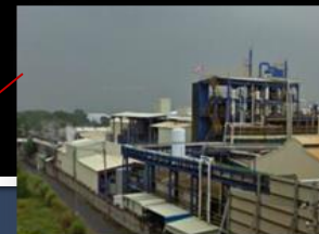
Ping Zhen plant 平鎮廠 -Agrochemicals 植物保護用藥 -Fine Chemicals 特用化學產品 -Clarifying agent 成核劑
