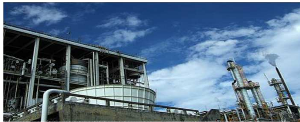
Taichung Relocation Plant
