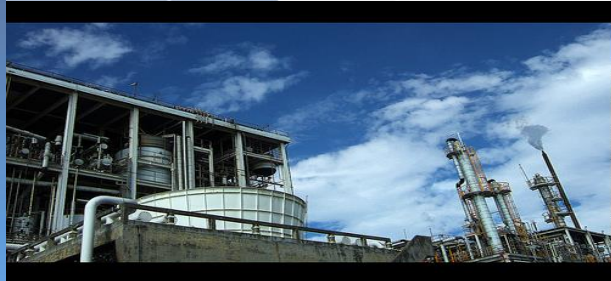
Taichung Relocation Plant
