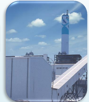
Roofing & Siding of Industrial Factory
