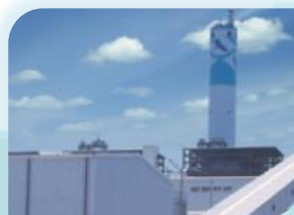
Roofing & Siding of Industrial Factory
