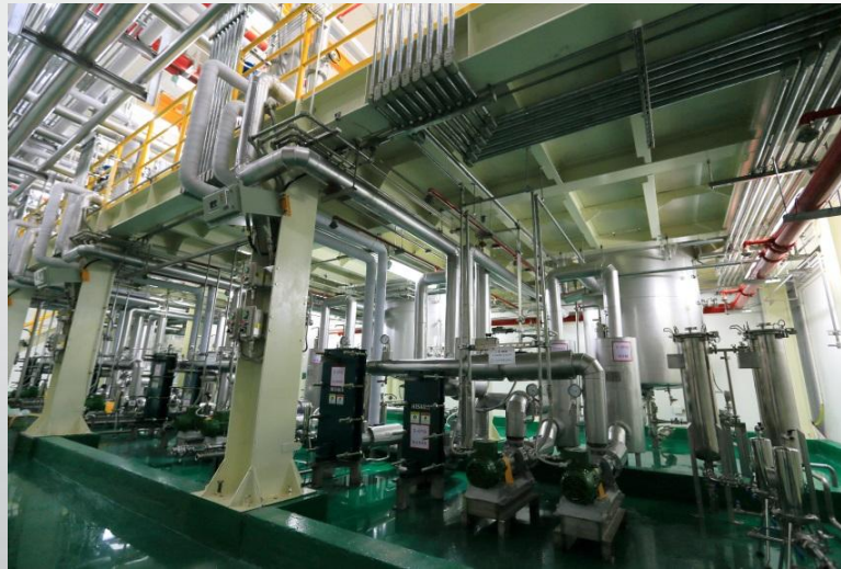
Stirring tank temperature control cycle
