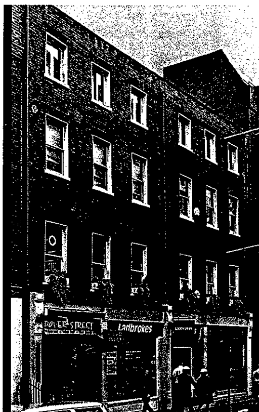
8/9 Dover Street, London W1
