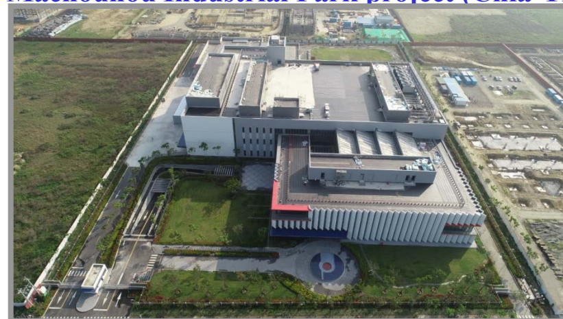
Machouhou Industrial Park project (Chia-Yi)
