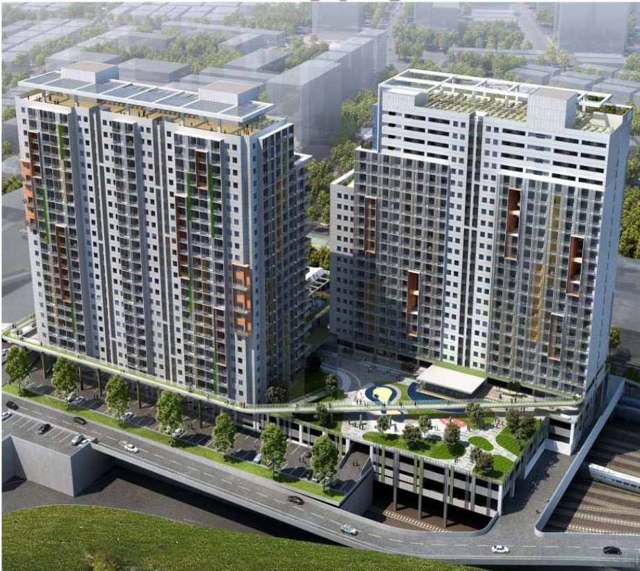
Nangang Depot Public Hopusing Turn-key project
