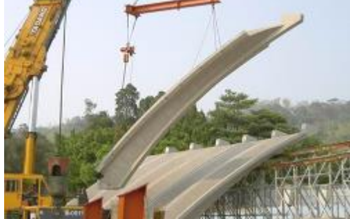
Prestressed Precast roof slab
