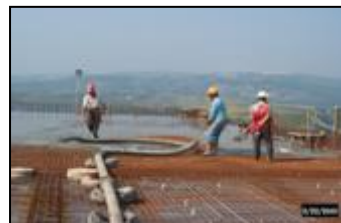
Reinforcement and concrete casting for floor
