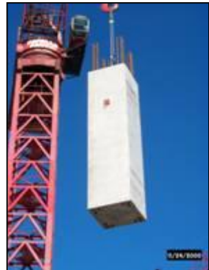
Column installation
