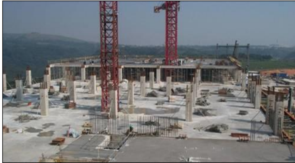
Reinforcement and concrete casting for floor
