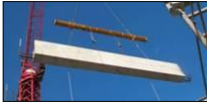
secondary beam installation
