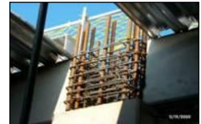
Reinforcement for Beam-column joint
