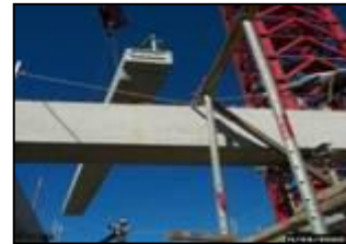
secondary beam installation
