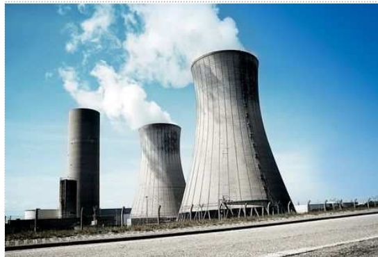
Nuclear Power Cabinet
