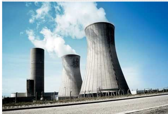
Nuclear Power Cabinet
