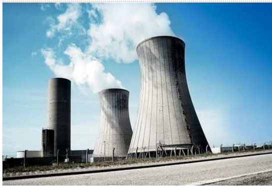
Nuclear Power Cabinet
