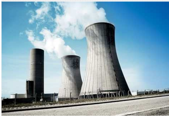
Nuclear Power Cabinet
