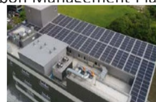
Solar Panels Implementation
