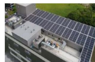
Solar power system installation
