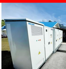
帛琉 PV 218.4kWp + ESS 200kW/1,720kWh
