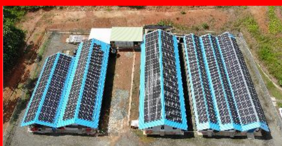
帛琉 PV 218.4kWp + ESS 200kW/1,720kWh
