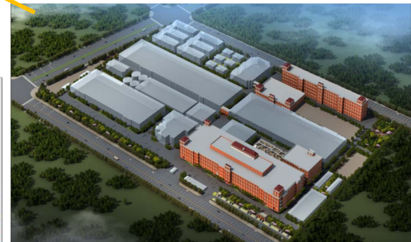
JiangSu- WuXi Site II (2007~)
