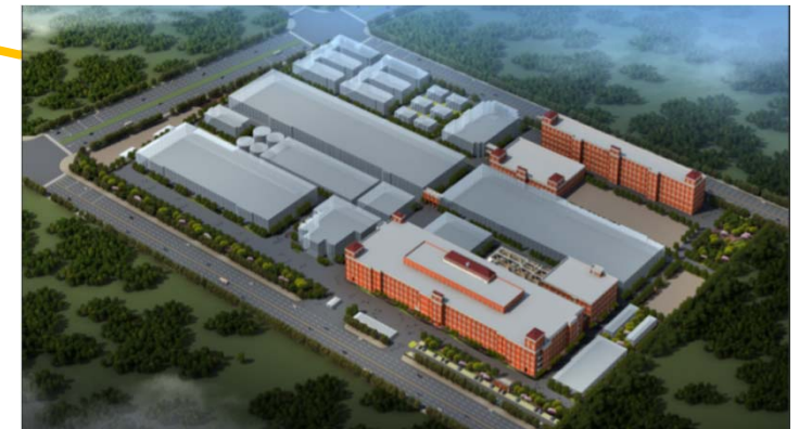
JiangSu- WuXi Site II (2007~)
