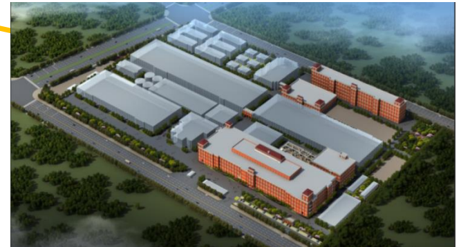
JiangSu- WuXi Site II (2007~)
