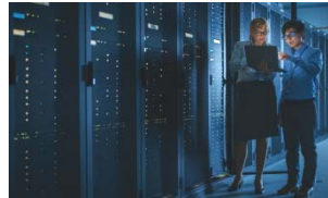
Mission Critical Power UPS
