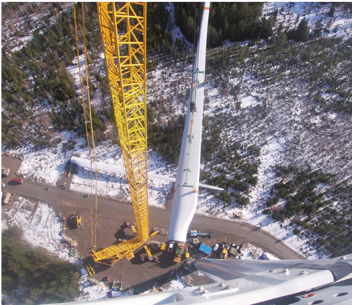
Ljungbyholm: Hoisting a blade into position
