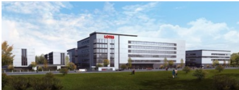
New plant in Zhongshan: 140,000 sqm
