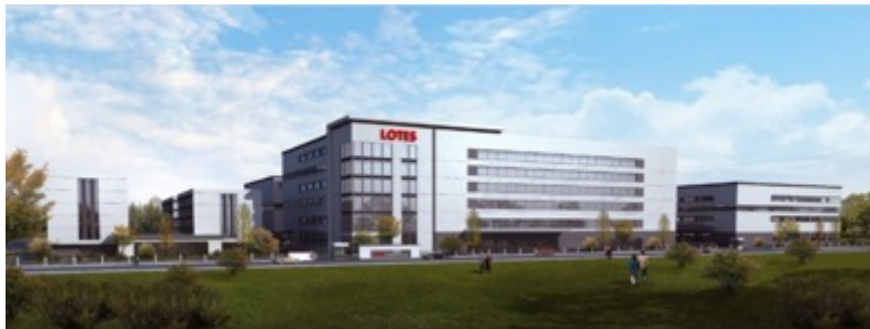
New plant in Zhongshan: 140,000 sqm
