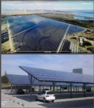
Large car park
