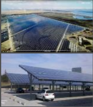
Large car park
