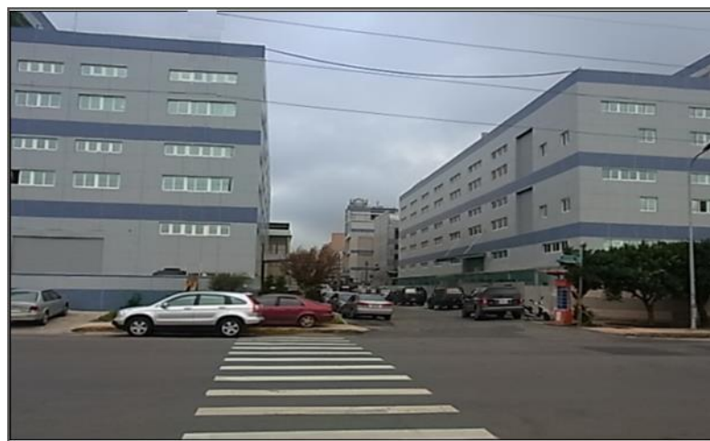
Taiwan, Dayuan Plant
