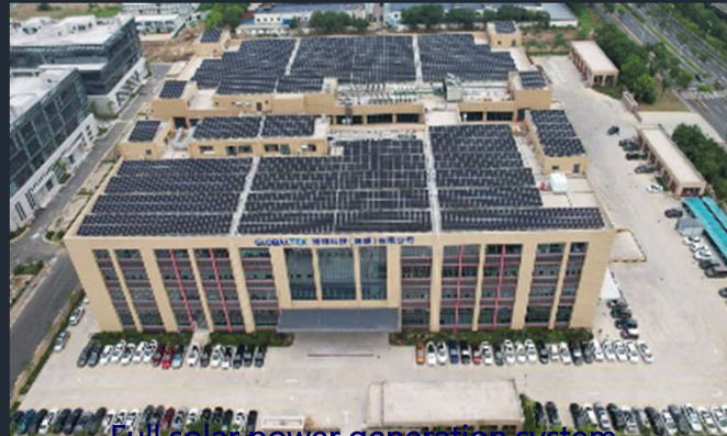
Full solar power generation system In Global Tek Wuxi, Jiangsu Province, China
