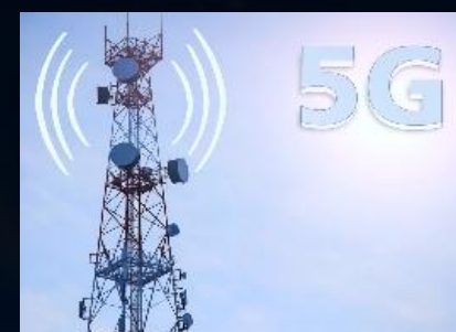
5G Network Equipment
