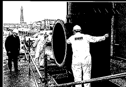
This 60-inch axial flow storm water pump and motor, one of eight built by Mather & Platt in 1964 for a major pumping station in Blackpool, was overhauled by Helysham service centre for North West Water.
