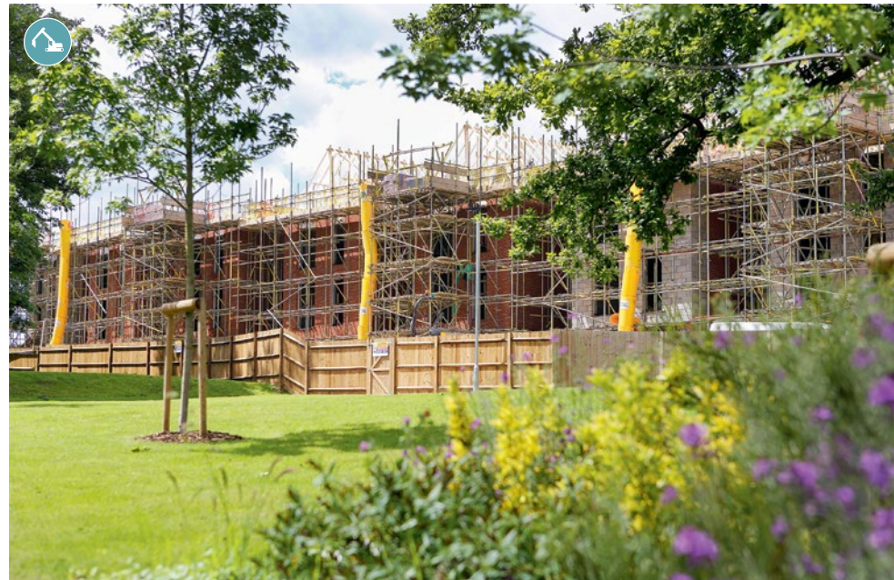
Cane Hill Park in Coulsdon, Surrey where we are trialling the use of Light Gauge Steel Frames in the construction of apartments and using timber frames in the construction of houses.
