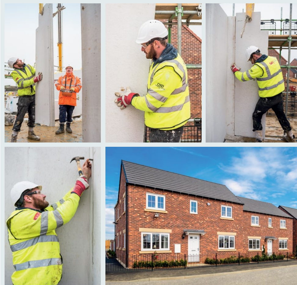
Large Format Block being used in construction at our Longford Park development in Banbury, Oxfordshire.
