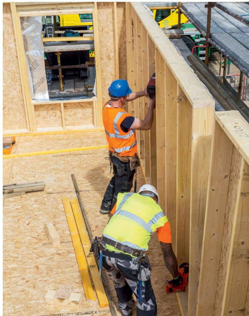
Timber frame external wall panels being fixed into place at our Osprey Heights development in Inverurie, Aberdeenshire.
