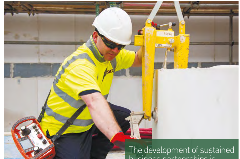
A crane driver from our partner SIG Roofspace Ltd attaching the clamp to the Large Format Block in readiness for lifting.
