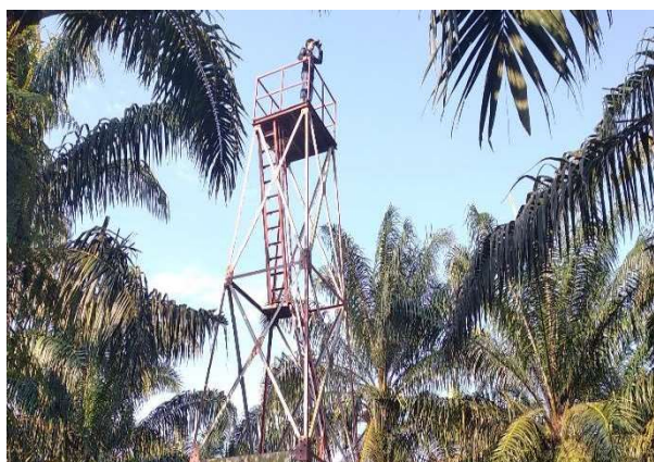
Monitoring hot spots from fire tower
