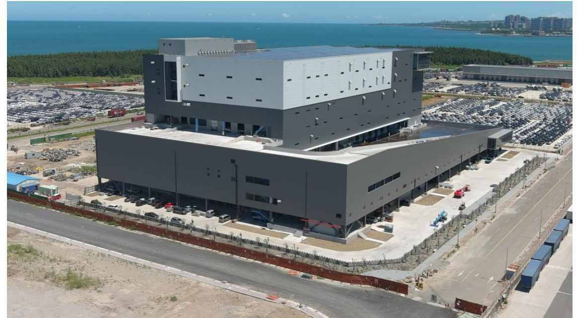
Phase I Warehouses - Aerial View
