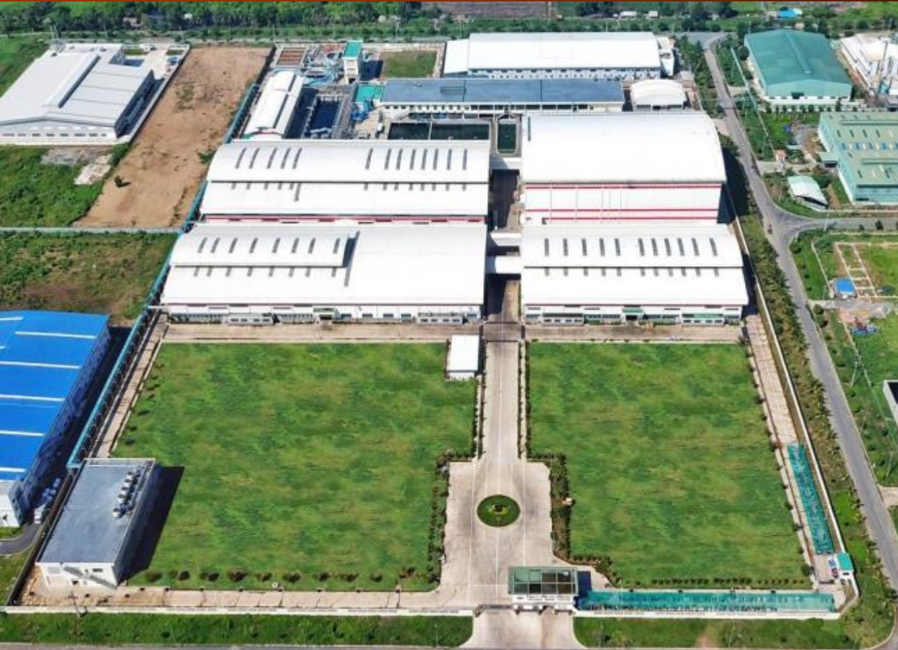
Vietnam Factory II (Le Minh Xuan 3 Industrial Park)
