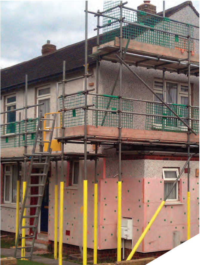
External wall insulation is fitted by our Affordable Housing division to improve building energy performance
