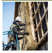
Many aspects of the development are being constructed using traditional methods and locally sourced materials including timber, straw and heather. 'Cassette cladding' – a completely new way of using thatch – is one of the key sustainable elements being incorporated into the build project. Developed by the University's Adapt Low Carbon Group and delivered by Construction &
