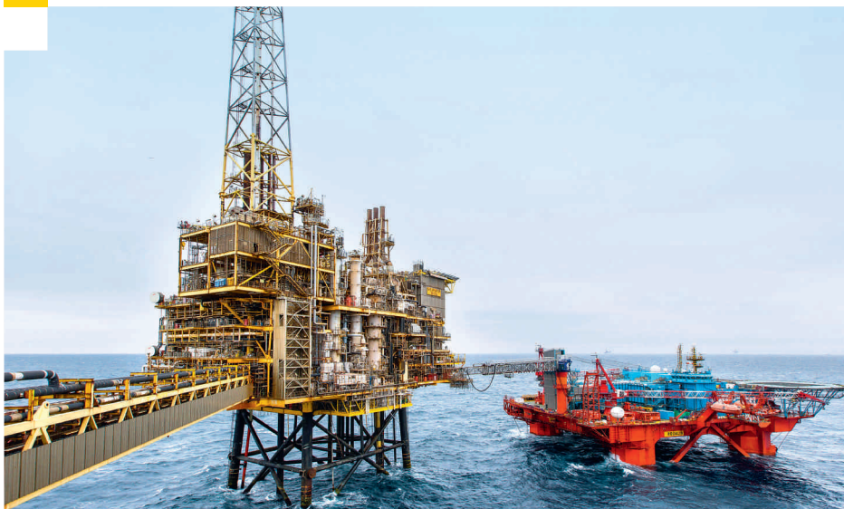
The Shearwater gas platform off the coast of Scotland in the UK North Sea.
