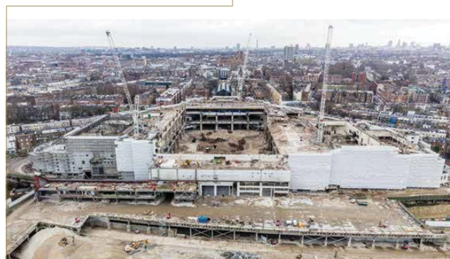
EC2 roof and structures demolished and the roof of EC1 demolished and removed from site
