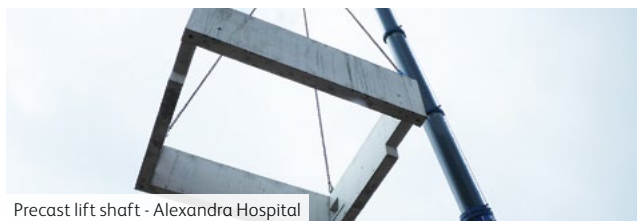
Precast lift shaft - Alexandra Hospital
