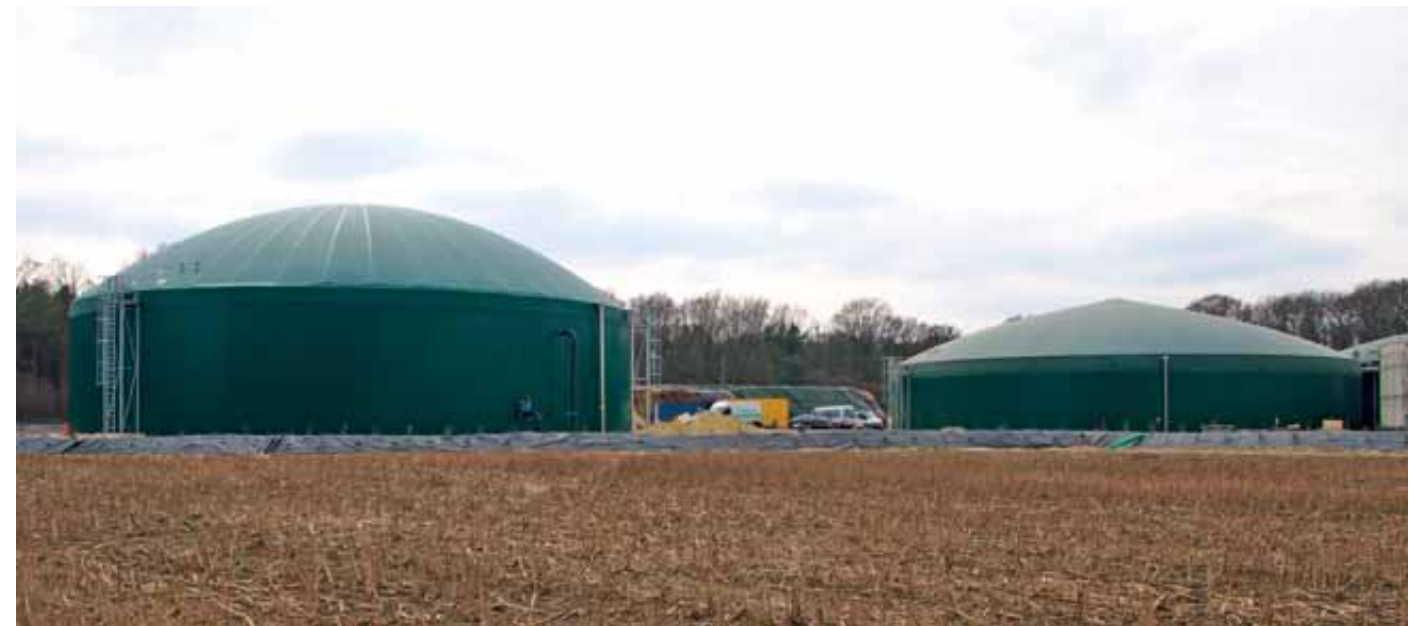
Making the good even better: The energy-carrier biomethane can be stored in considerably greater volumes with double membrane roofs.
