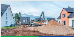
START OF CONSTRUCTION
