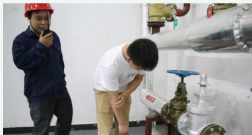
Emergency Exercise for Steam Pressure Pipeline Leakage
